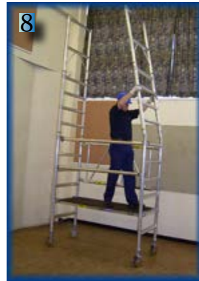
Interlock Clip unlocked
